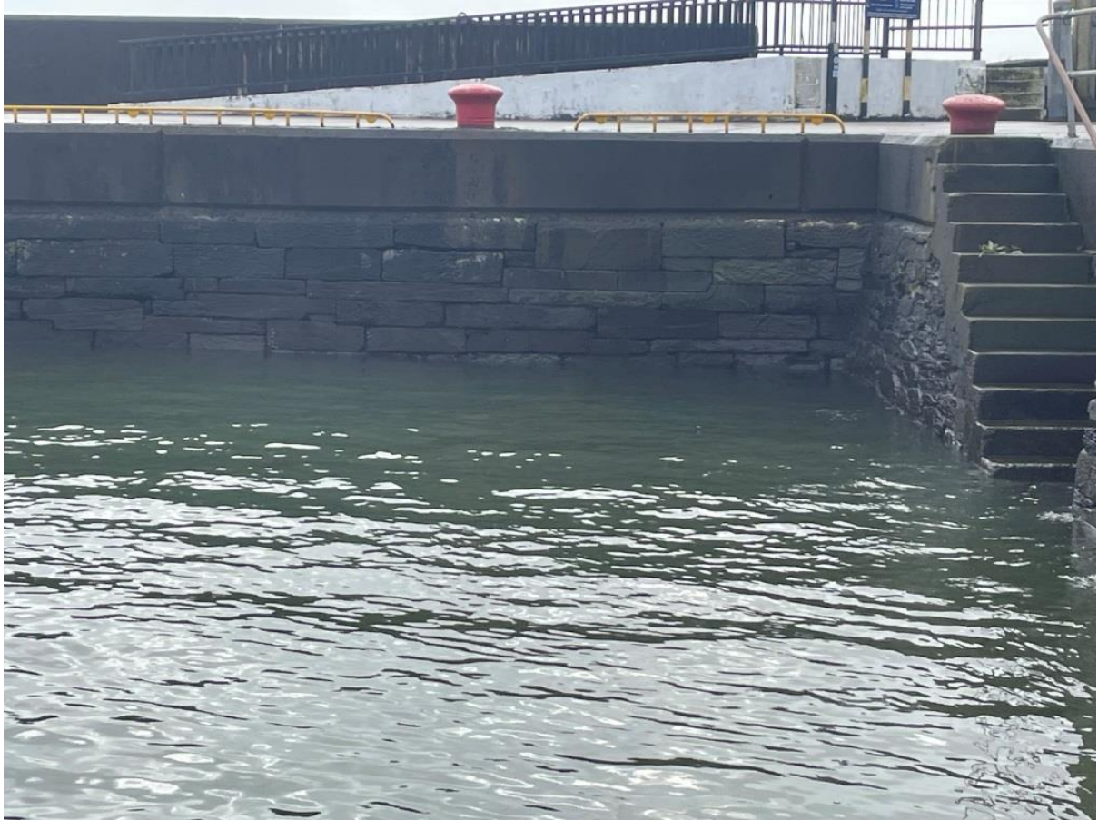
Schull Pier Pontoon – Photographs 03.2026
