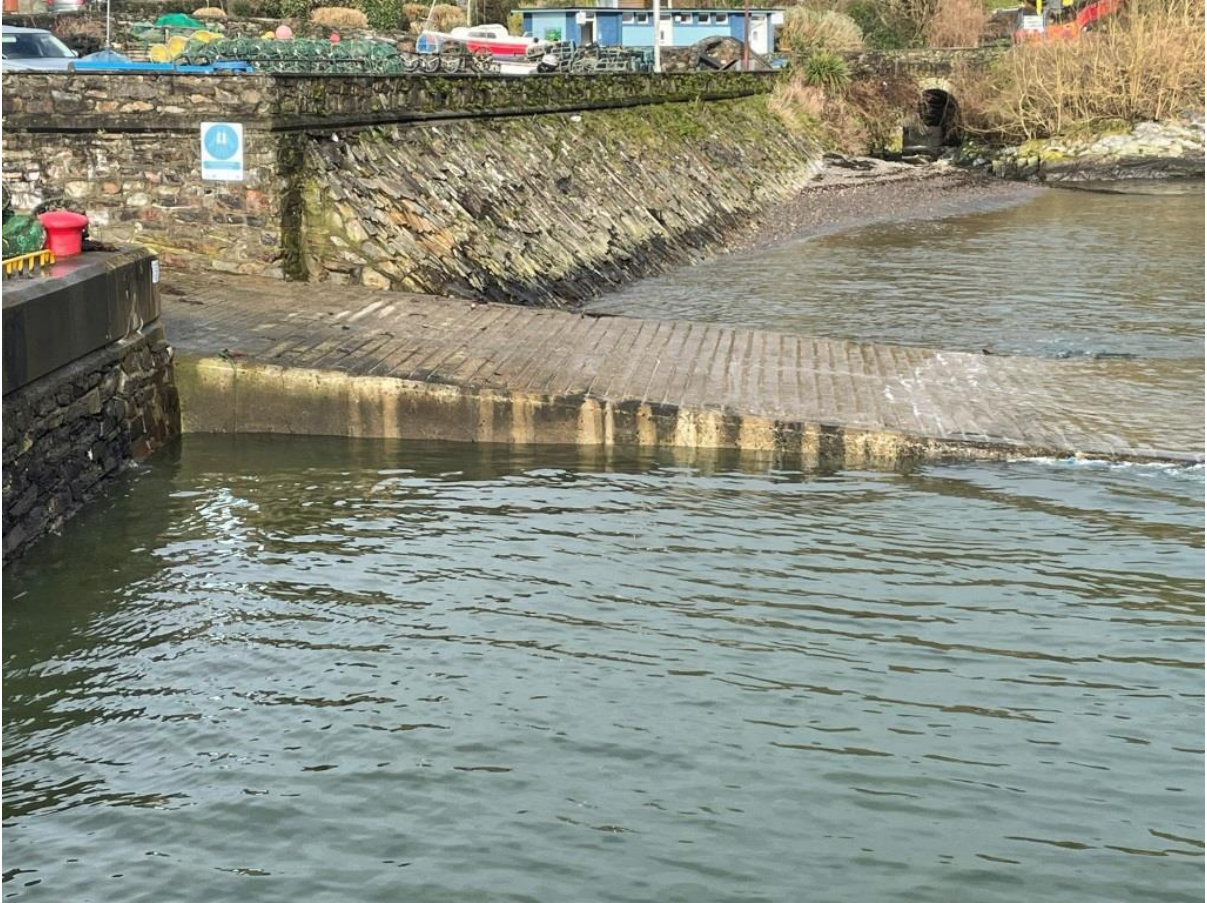
Schull Pier Pontoon – Photographs 03.2026
