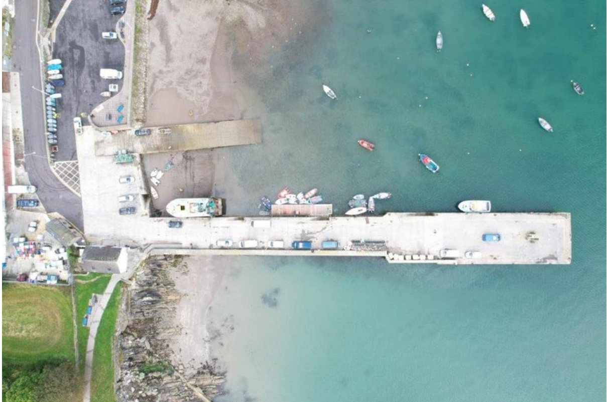
Schull Pier Pontoon – Photographs 03.2026
