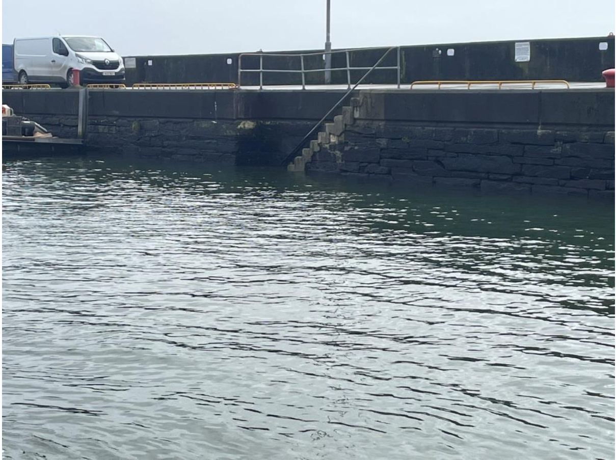
Schull Pier Pontoon – Photographs 03.2026
